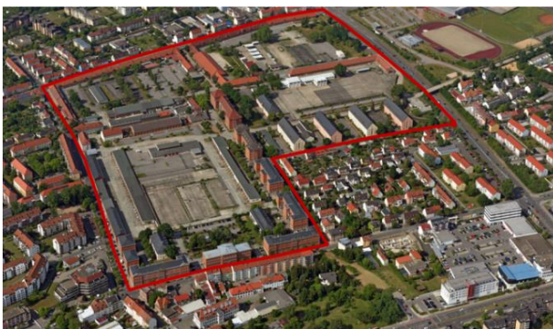
Figure 1 Aerial view of the former Lagarde barracks [1]
